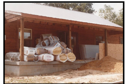
The Manna House getting closer to completion (around 1983).
